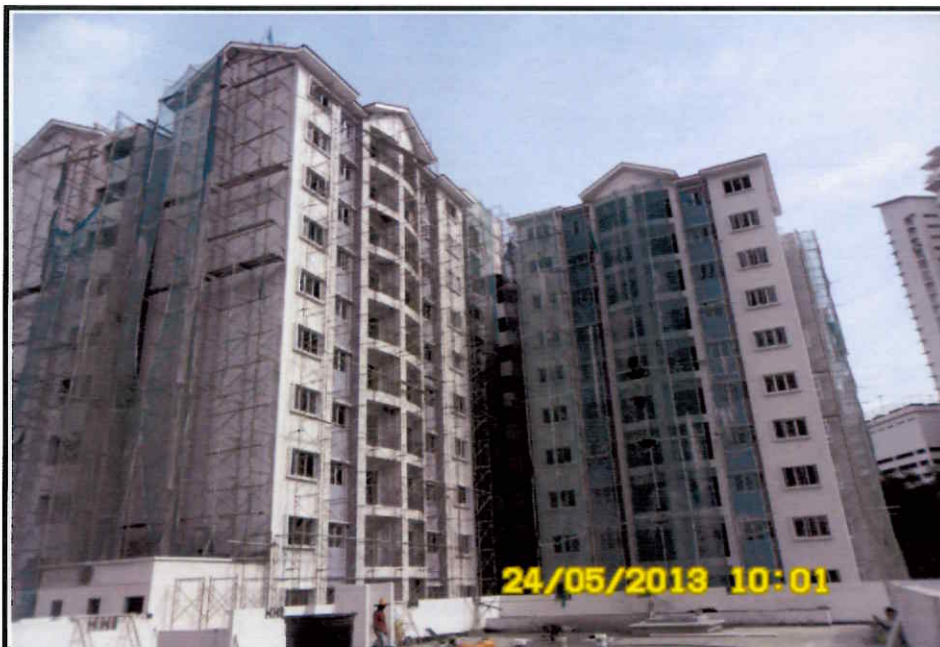
External elevation view of Block A as of 29/05/13
