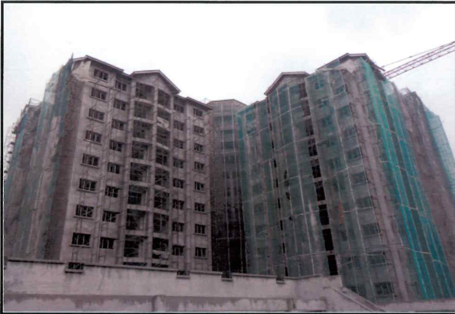
External elevation view of Block A as of 14/03/13
