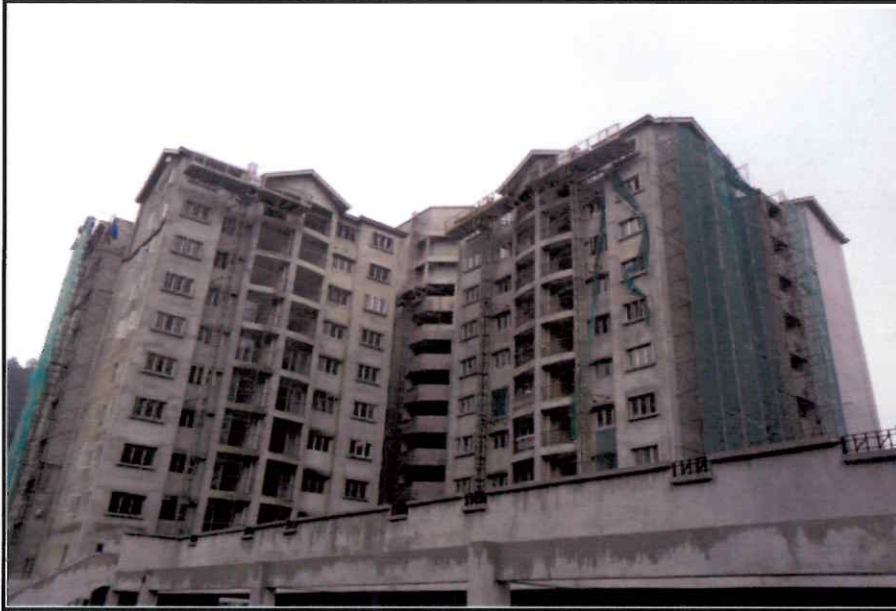
External elevation view of Block B as of 14/03/13
