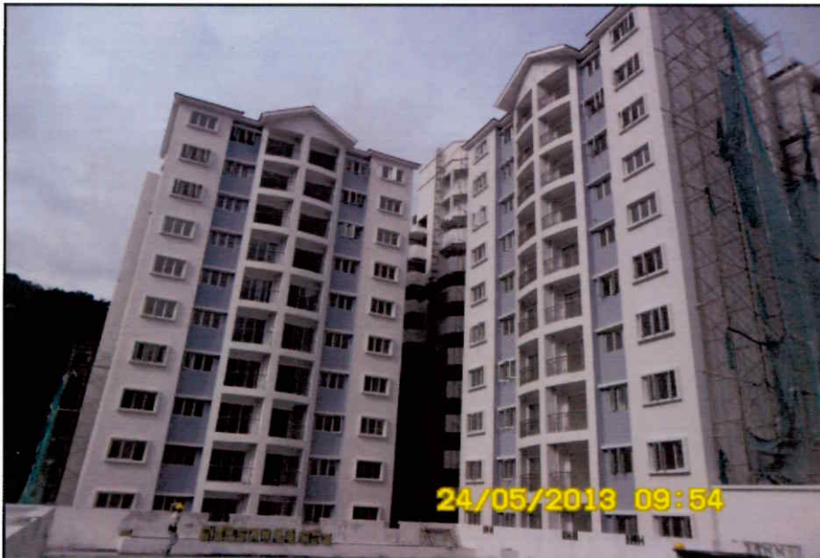
External elevation view of Block B as of 29/05/13
