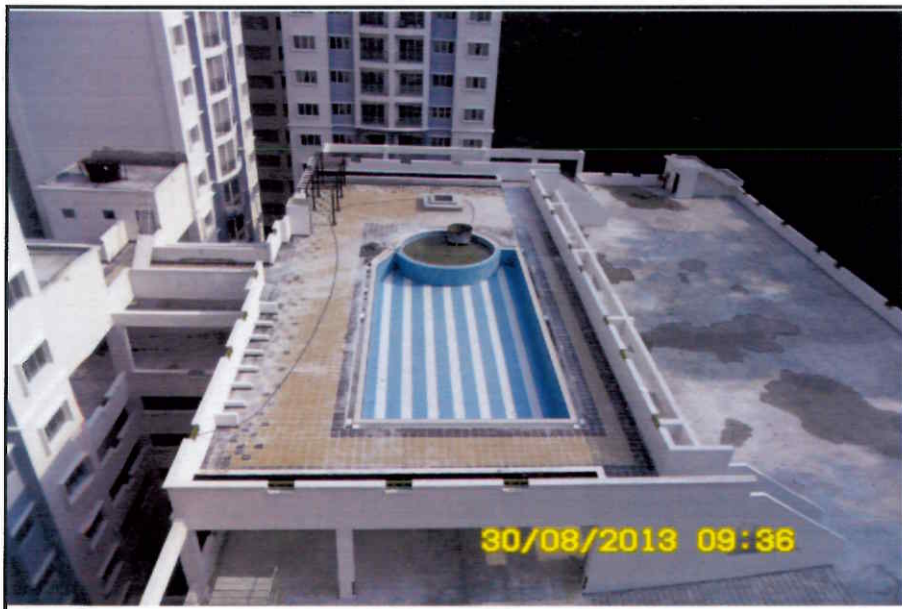
External view of swimming pool as of 29/08/13
