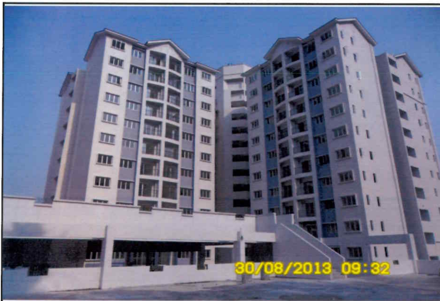
External elevation view of Block B as of 29/08/13
