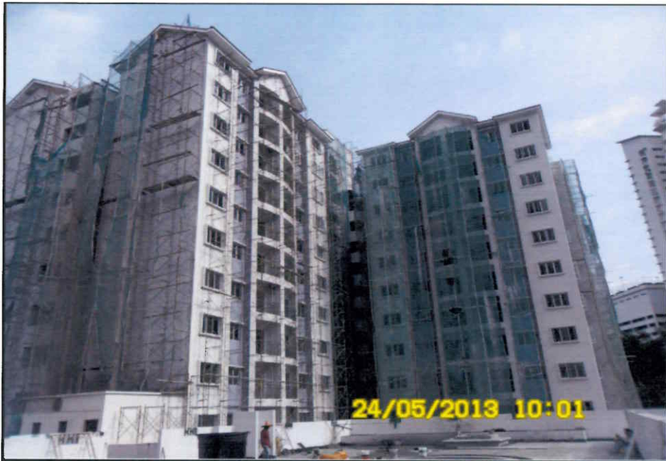
External elevation view of Block A as of 24/08/13
