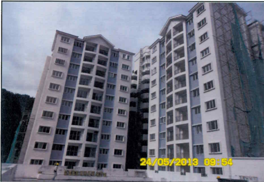
External elevation view of Block B as of 24/05/13
