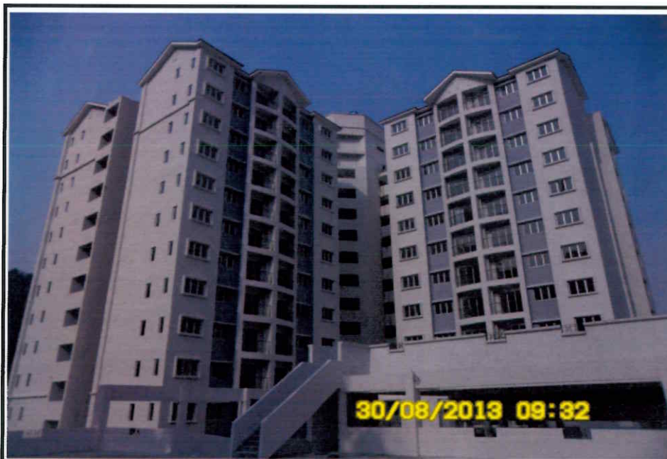
External elevation view of Block A as of 30/08/13
